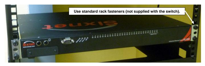
The above image shows an EL228 in reverse/rear style arrangement (ports and power in the back)
